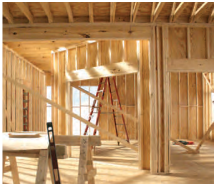
NEW HOME CONSTRUCTION
